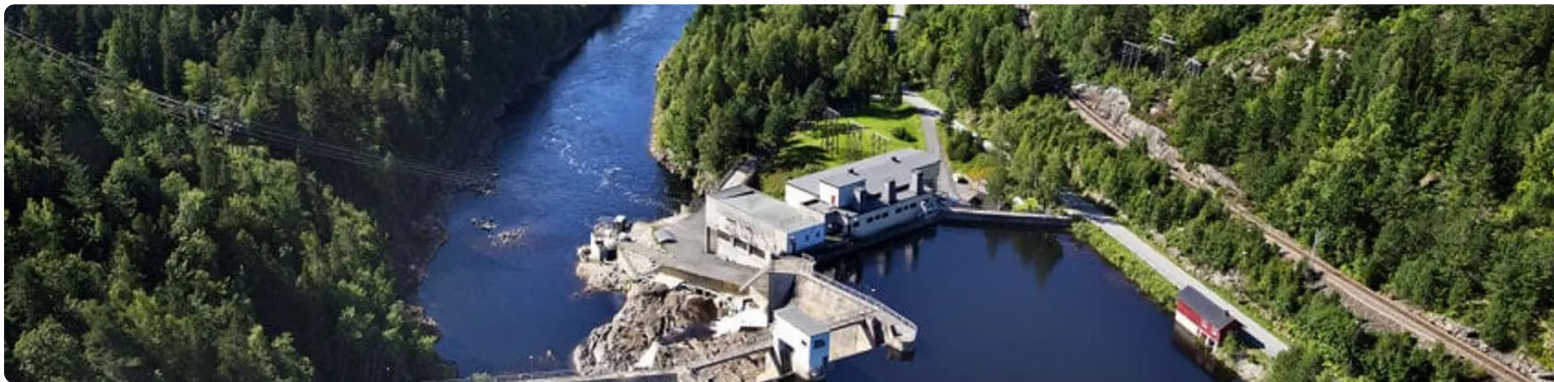
Evenstad hydropower plant.
